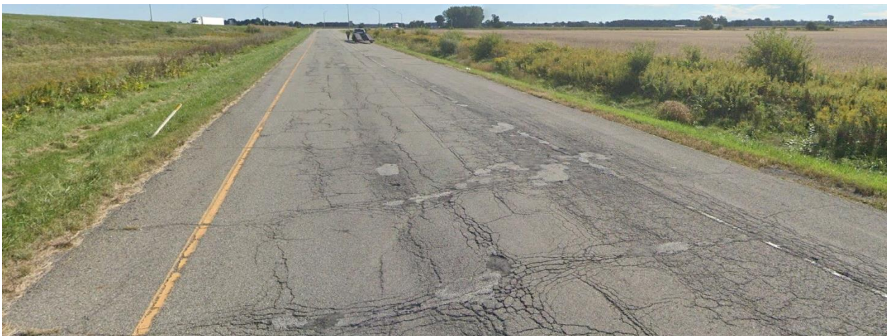
Figure 6 – US 35 Ramp Pavement (Sept 2022)
